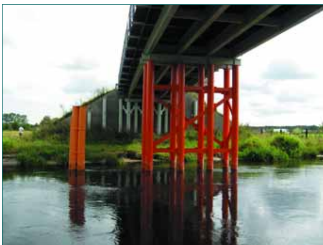
Major bridge structure on the Pisa River at PL-10.
