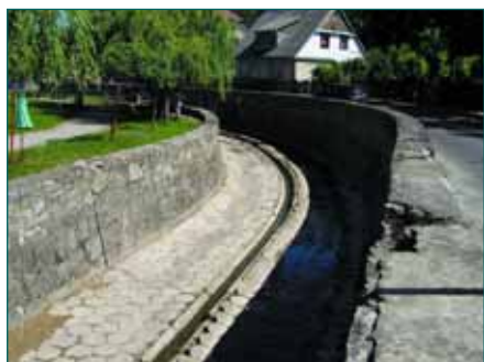
Artificial reprofiling and reinforcement of banks and the channel produce a high HMS score.
