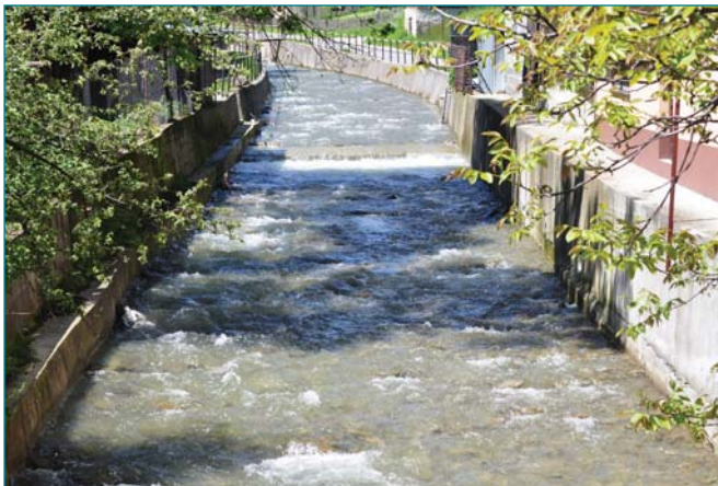
Concrete banks-an extreme form of channel modification.
