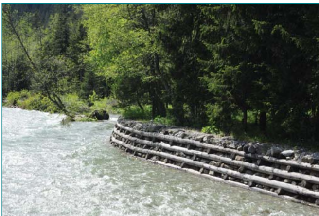
Tree trunk and boulder bank revetment.
