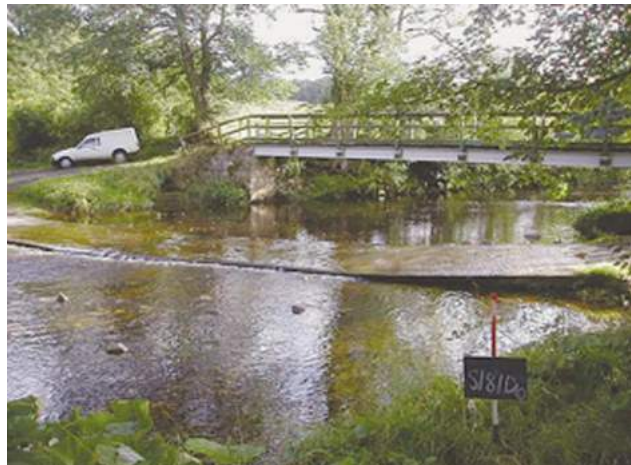
D3f Minor bridge – bridge lacks in-channel supports and has bank abutments <10m wide. Note major ford in fore-ground.
