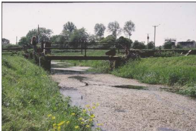
Na Realigned channel choked with submerged aquatic vegetation. Note minor bridge. See also A1b. Do not record 'channel choked' when just free-floating vegetation (see A3b).
