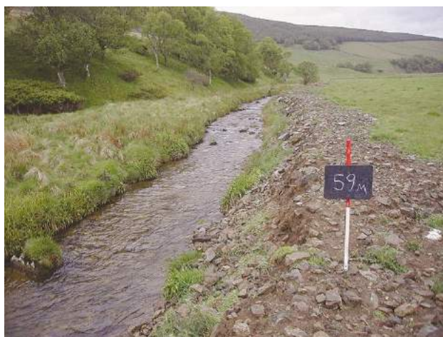
E6f Resectioned channel – this shows a mobile, gravel-bed, river that has been resectioned, with tell-tale spoil on the right.
