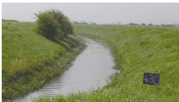
E6e Resectioned bank – this example shows river with few trees, very even gradients to the banks, and with the banktop width <4 times the banktop height indicating both deepening and resectioning.
