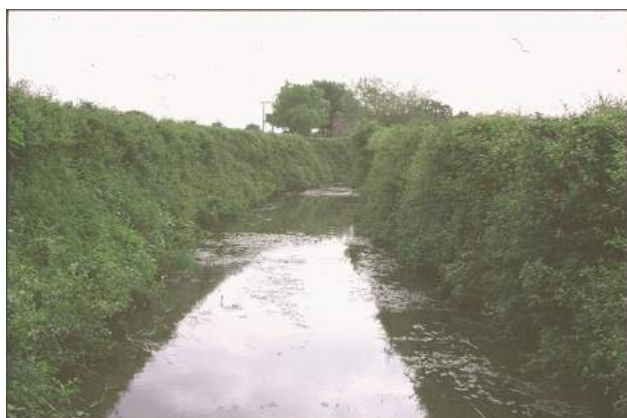
D8a Over-deepened channel – very obvious tell-tale signs are the uniformly sloping, artificially steep, banks and a channel width/bank depth ratio <4:1 . See also E2Aa.
