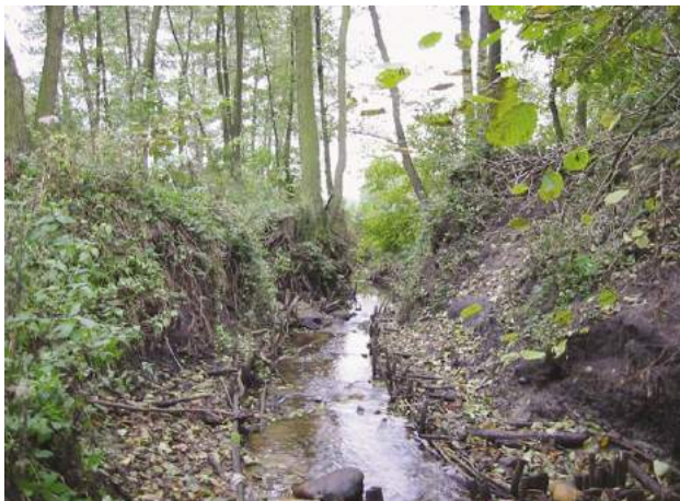
E1Pc Bio-engineering bank materials – woven dead stakes and twigs.
