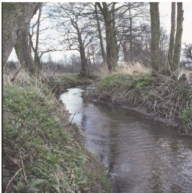
E6a Resectioned channel – typical signs seen here include deep channel cf. width, steep smooth-sloped banks, and even-aged trees only on top of bank. See also A1a-c, I6b.
