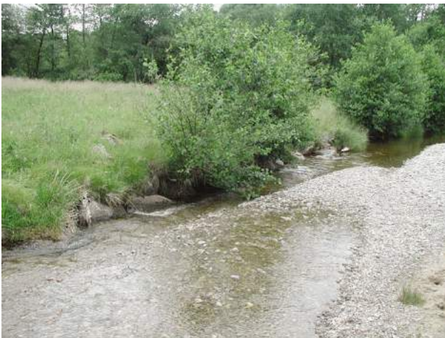
I6a Reinforced bank – toe only; reinforcement is with large boulders (rip-rap). See also E1Ja,b, E1Ka, E1Oa.
