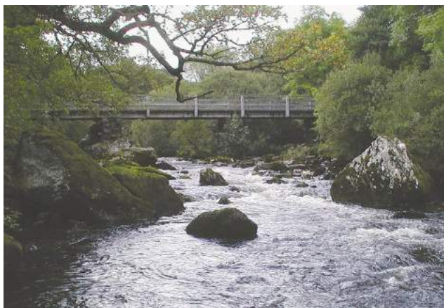
D3e Minor bridge – pipelines crossing rivers, if lacking central piers, are recorded as minor bridges. See also Na. Note exposed boulders and broken standing waves.
