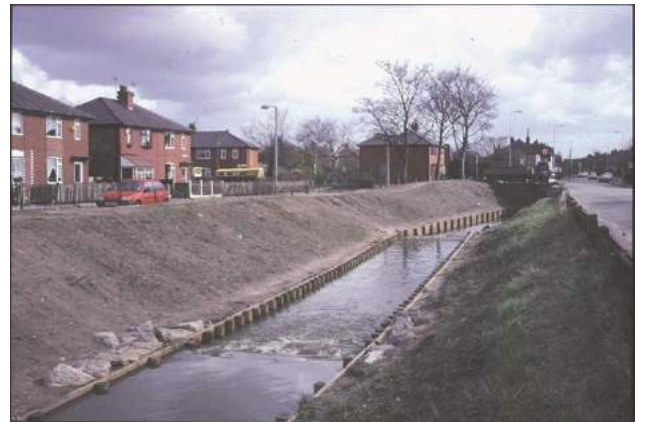
I6b Reinforced bank – toe only; reinforcement is wood-piling. Note also bed and banks have been resectioned, and a series of low weirs installed.
