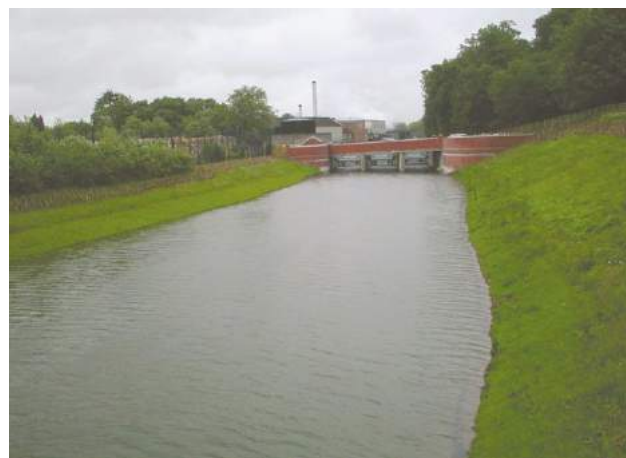
E2Ab Resectioned (reprofiled) bank – tell-tale even (trapezoidal) slope of newly resectioned bank.
