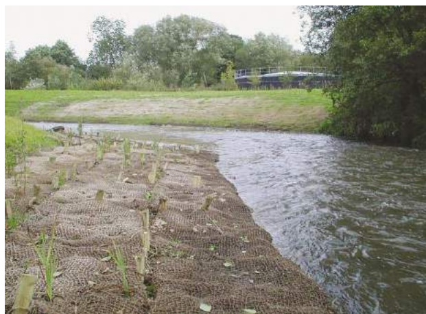
E1Pa Bio-engineering bank materials – bio-degradable matting with vegetation planting. Record bank vegetation structure as 'bare'.
