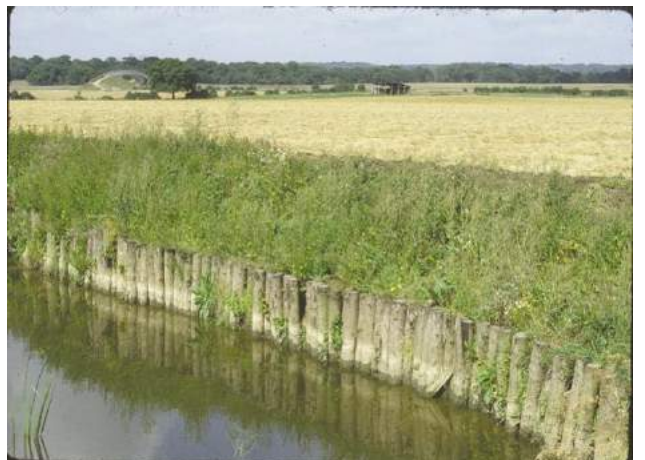
E1Jb Wood piling bank material – vertical poles below resectioned bank and arable (tilled) land-use in background.
