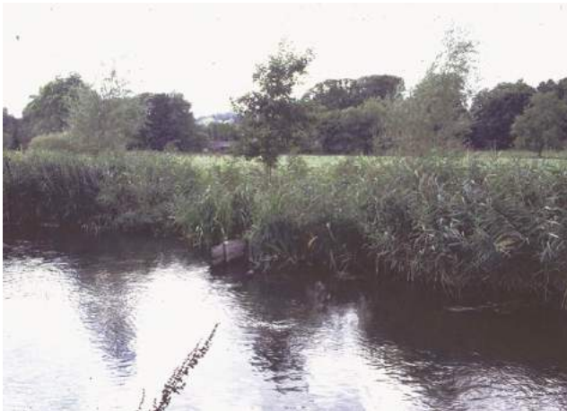
D6e Minor deflector/groyne/croy – extends across <10% of the channel width (installed to encourage reed encroachment that now almost obscures the deflector).
