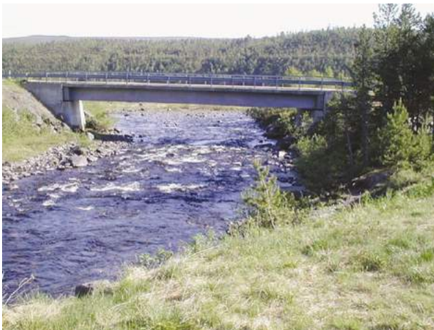
D3c Intermediate bridge – no central piers, and with bank-side abutments 10-25m long. Note broken standing waves.
