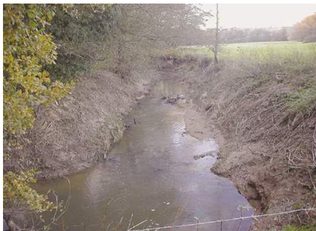
D8b Over-deepened channel – obvious signs include the slumping of the artificially steep banks and the channel width/bank depth ratio is <4:1 .
