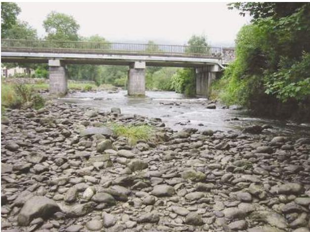
D3a Major bridge – all bridges with central piers are classed as 'major'. Note importance of photographs to show size of piers, and degree of associated bed armouring. Classic cobble channel substrate exposed in foreground. See also D5b.
