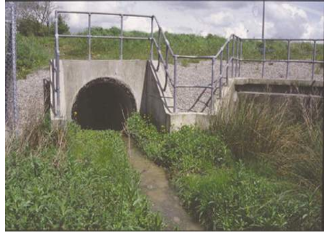
D2a Culvert – all are recorded as 'major' structures. When channel modification records 'CV', and it is impossible to see the bed and banks clearly, all other channel characteristics should be recorded as 'NK' or 'NV'.
