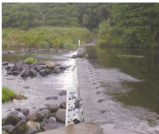
D5a Major ford – both the bed and banks are made of artificial material, and there is obvious ponding of water upstream. See also D3f.
