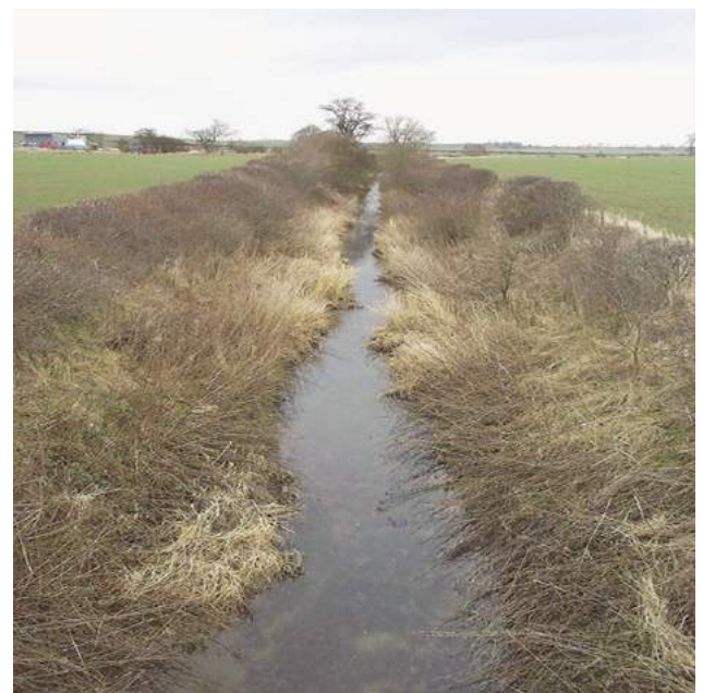
D7a An obviously realigned and over-deepened channel. Note hedge at the top of the bank that should be recorded as complex banktop vegetation structure.
