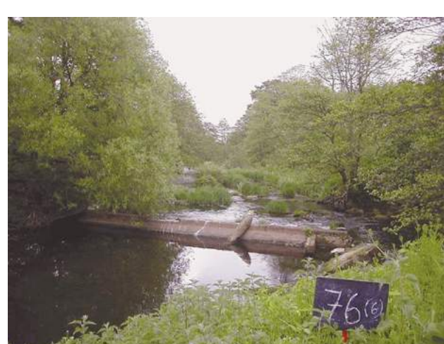
D6b This collapsed weir is recorded as a major deflector as it extends >20% across the channel.
