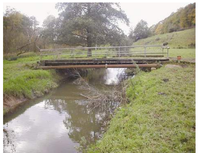
D3d Minor bridge – farm track bridges <10m wide are recorded as 'minor'.
