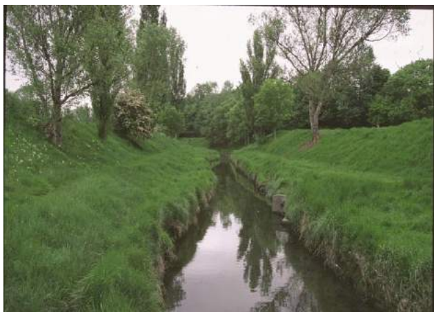
E2Ca Artificial Berm – formed by excavating bank material (here on both sides) to form a two-stage channel. Both the flat base of the berm, and the face of the top of the bank, constitute 'bankface'. See also E1Hb, F18b.
