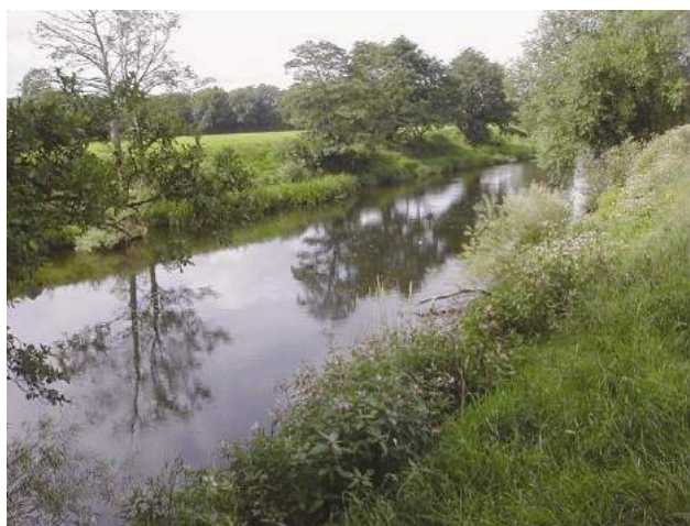
E6c Resectioned channel – even after many decades, past resectioning obvious due to even gradient of bank. Note also Himalayan balsam on near bank.
